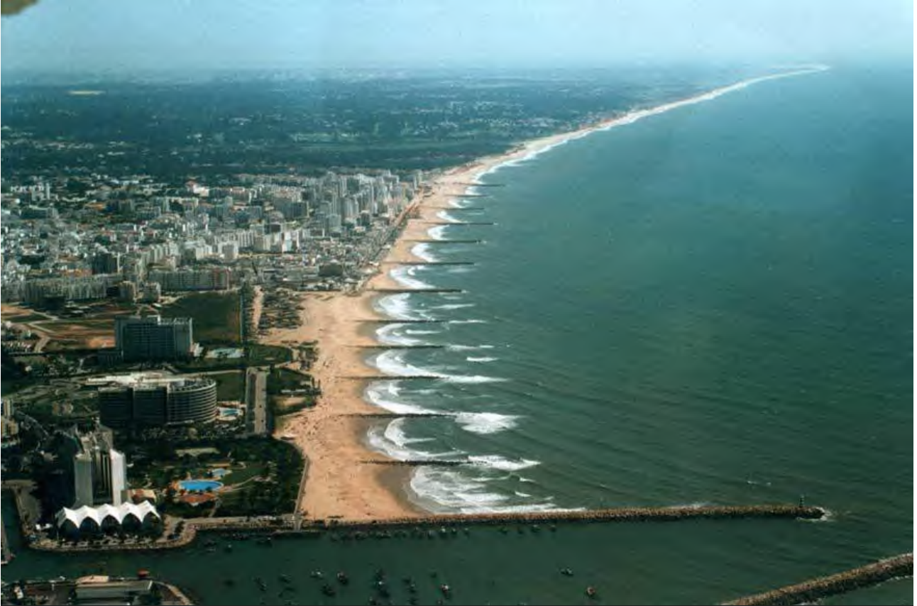
Figure 3.4: Groyne Field example, Australia
