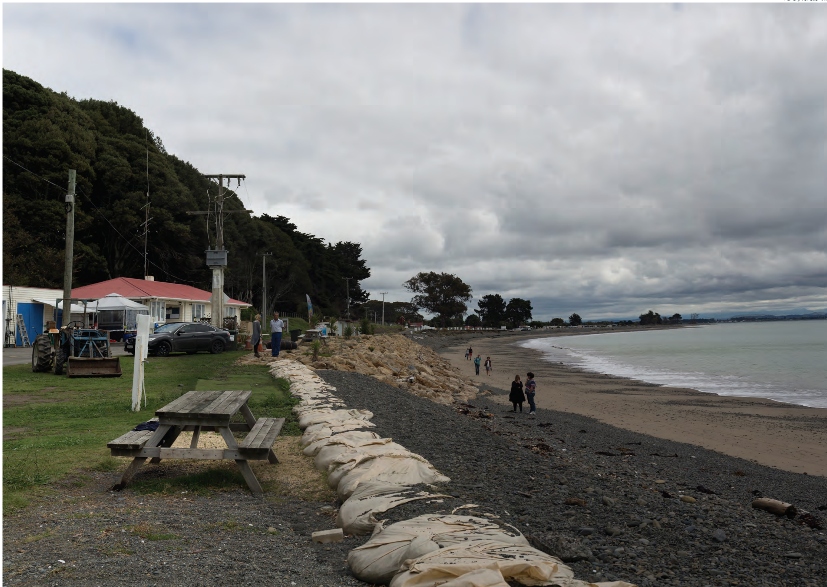
Clifton Motor Camp facing West towards existing sea defences and revetment.
