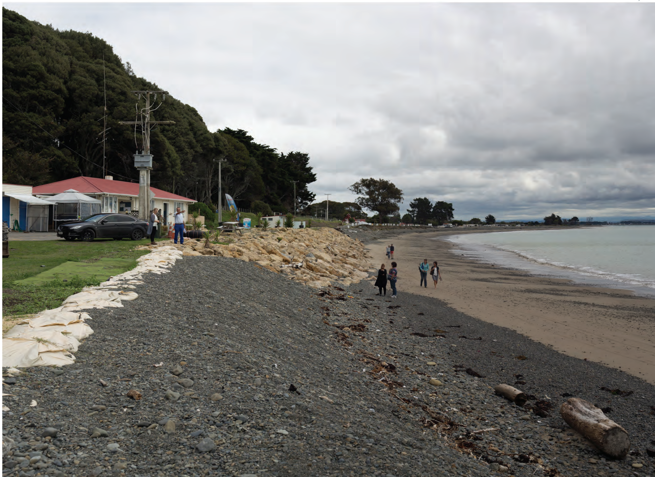
Clifton Motor Camp facing West towards existing revetment.
