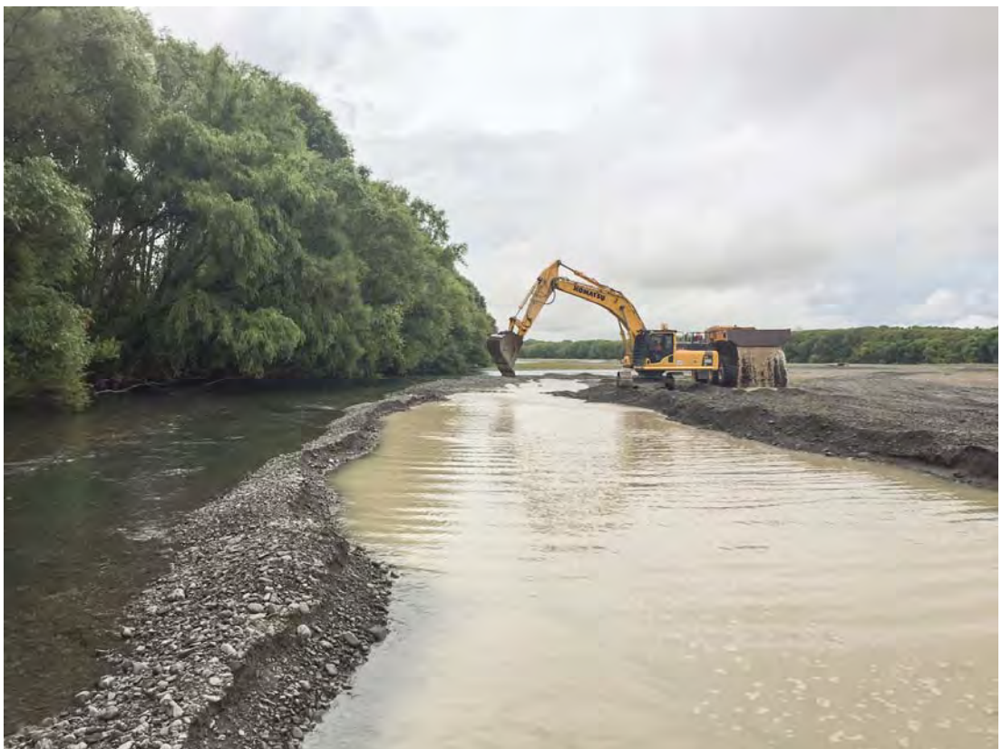
Figure 14: Typical gravel extraction operations showing works banded from main river on far left (adjacent to willow trees).
