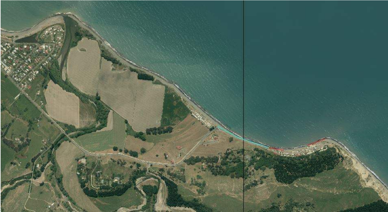
Figure 3.3: Hard point and Revetment Positions (red) and proposed revetment (cyan)
