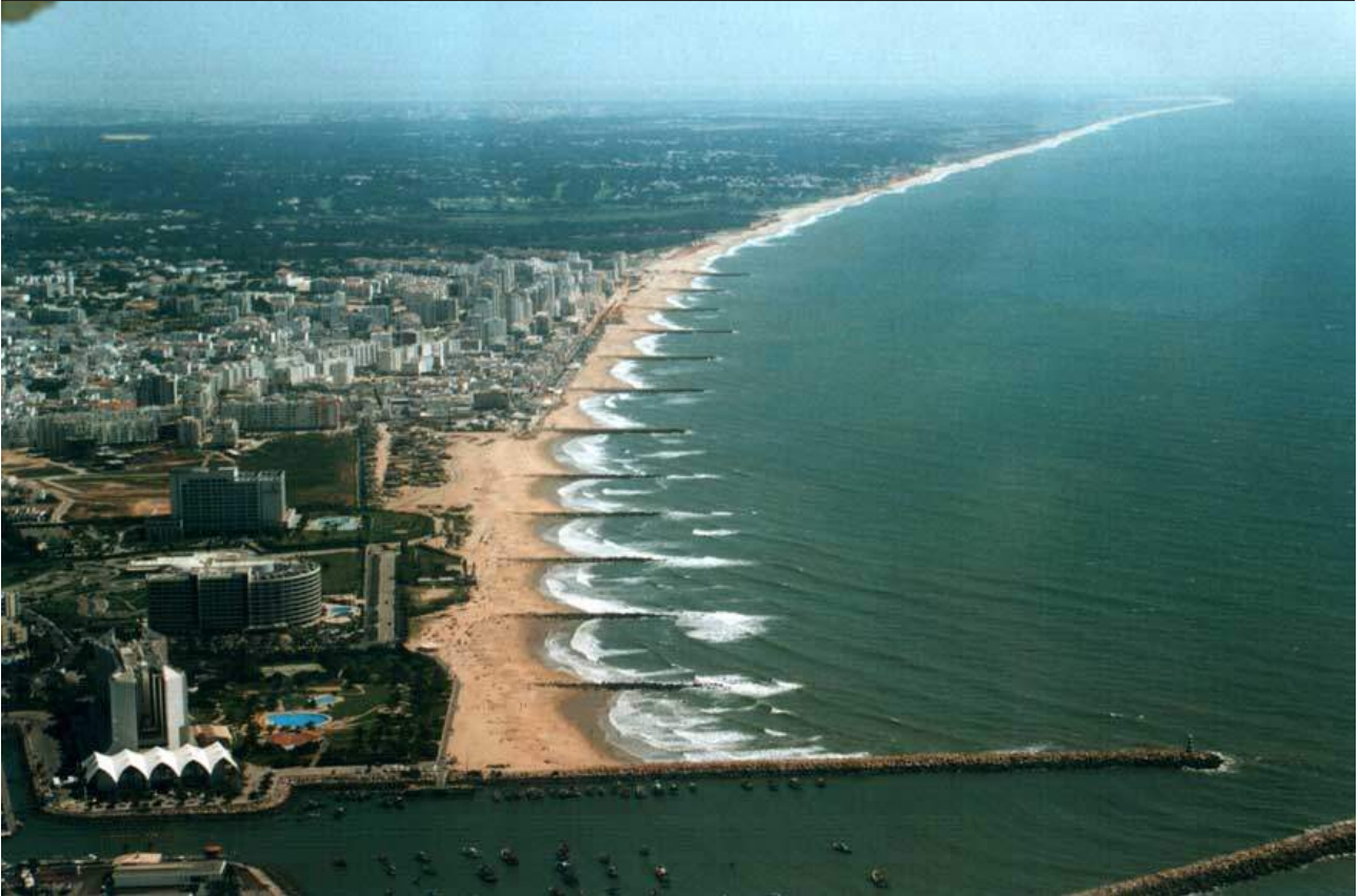
Figure 3.4: Groyne Field example, Australia
