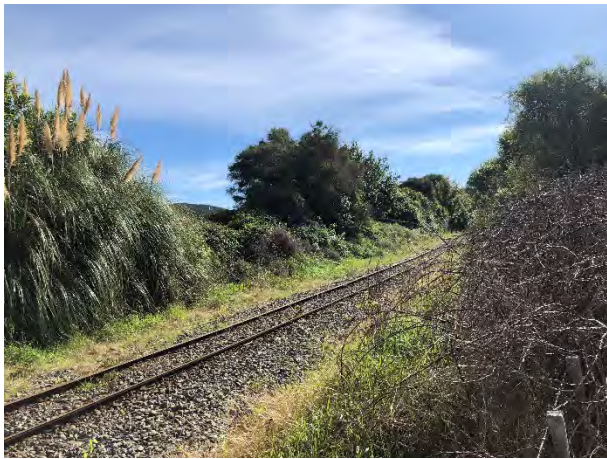
Plate 3-17: Pampas, blackberry and bracken weeds along the rail corridor provides skink habitat
