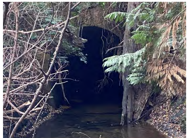
Plate 3-34: The stream is piped beneath Putorino Station Road, the railway line and a farm track
