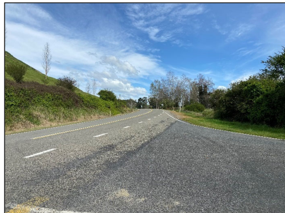
Figure 2.6: SH2 / Putorino Station Road Intersection - looking west towards SH2
