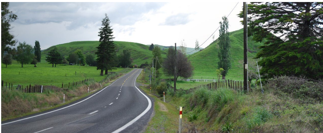
Fig 2.2b: Viewpoint 1: Representative view looking north east from the southern extent of the new alignment.
