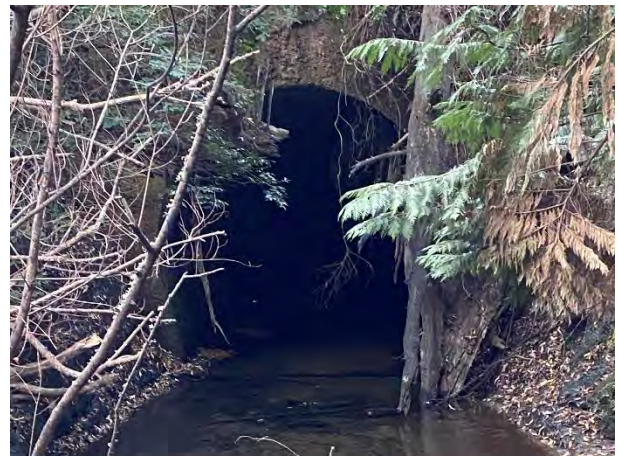
Plate 3-34: The stream is piped beneath Putorino Station Road, the railway line and a farm track
