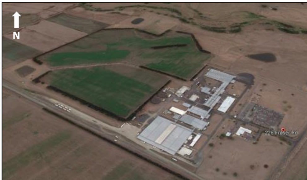
Figure 3: Takapau plant (Google Earth image)
