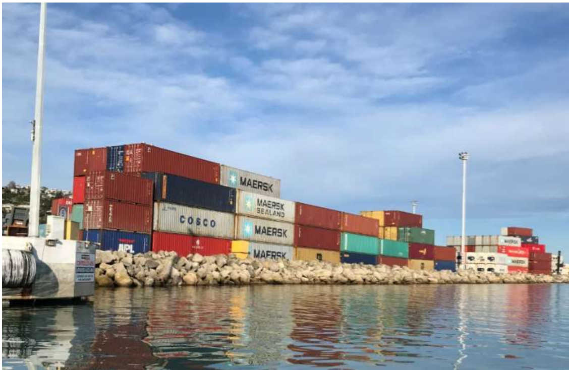
Figure 6. Existing Revetment 75 (site of proposed wharf)
