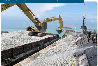
However if the outreach of the excavator is limited, there is an inherent possibility that the dredged material will drift and re-enter the excavated area. Loading excavated material into barges for transport remains the most common means of disposal.
