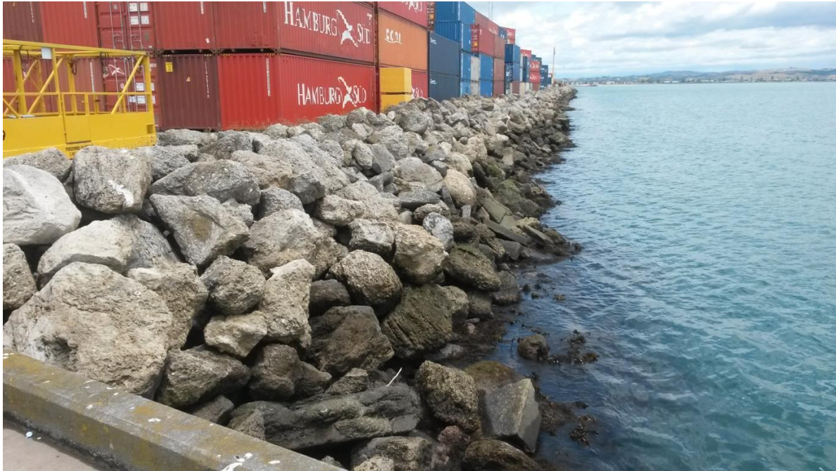
Figure 13-1: Existing revetment adjacent to proposed wharf
