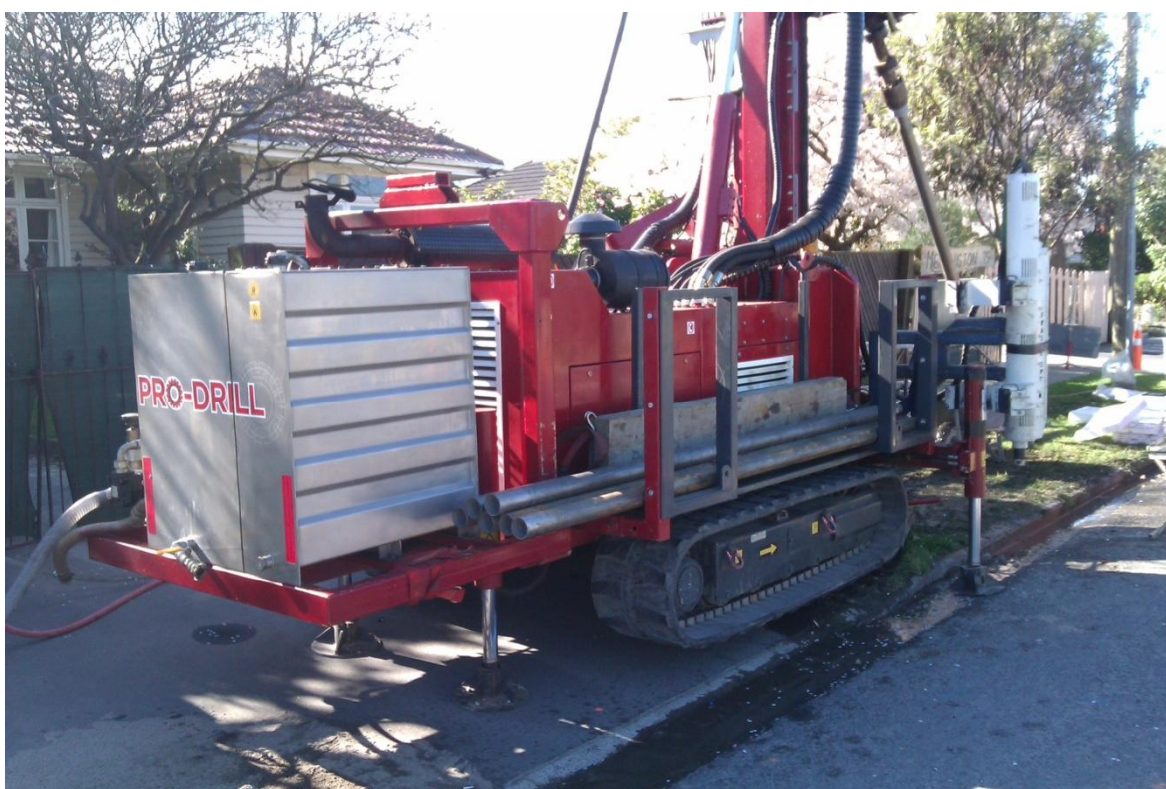
Figure 1. Track mounted Sonic drill rig "FRASTE1" with automatic SPT hammer
