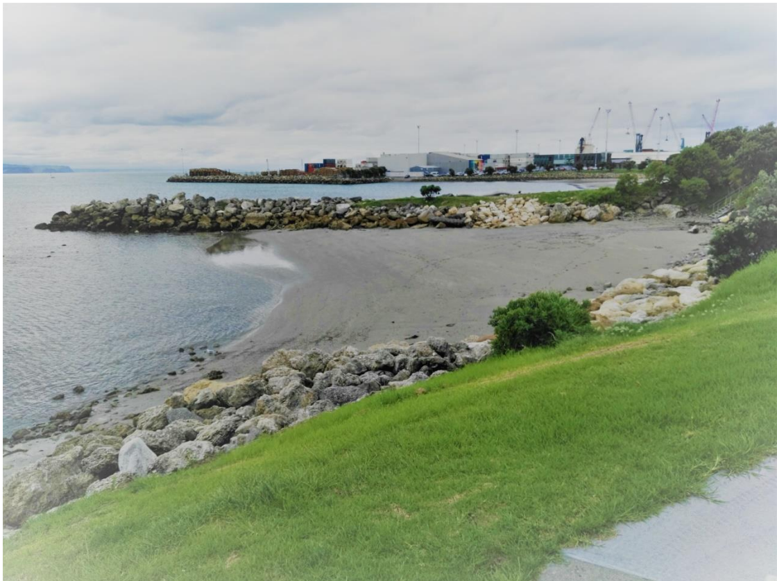
Plate 2: Limestone seawalls along the western edge of Napier Port (distance), around two small bays, including a groyne (centre), and along Hardinge Road (foreground). Pedestrian and cycle path is visible in bottom right corner.
