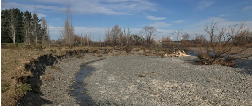
Figure 30: Waipawa River erosion upstream of SH50 Bridge
