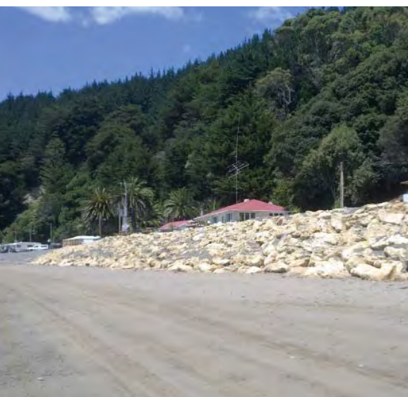
Completed limestone rock seawall
