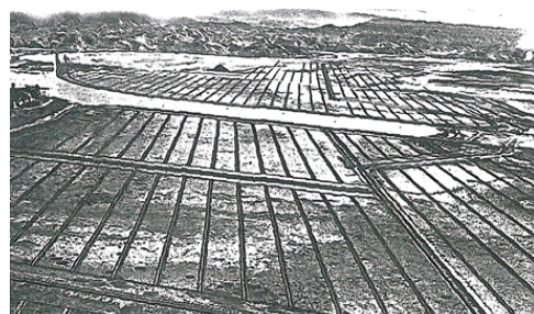
Tile drains were created in place of the exposed lagoon bed, after 1931
