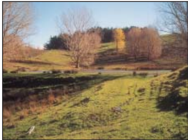
A well sited dam. Note: the well grassed spillway in the foreground.
