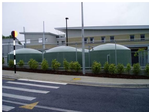
Water Reuse at a Hospital Site
