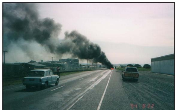
*Burning on the road surface to remove excess tar.*
