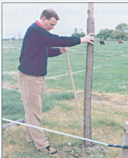
This Netlon protected pole is being re-rammed correctly. Ram at an angle and about an inch out from the base of the pole to ensure the pole is not damaged.
