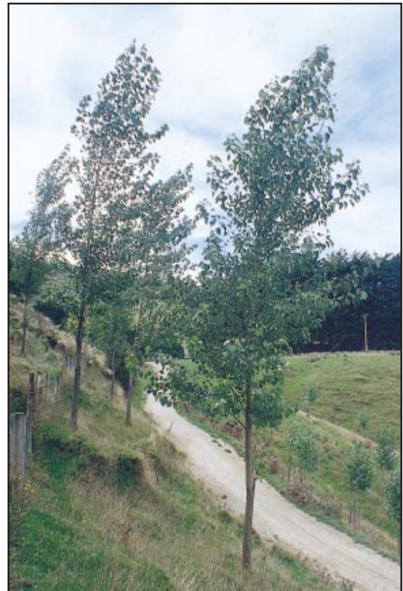
Poplar poles used to stabilise slopes above and below a farm track.
