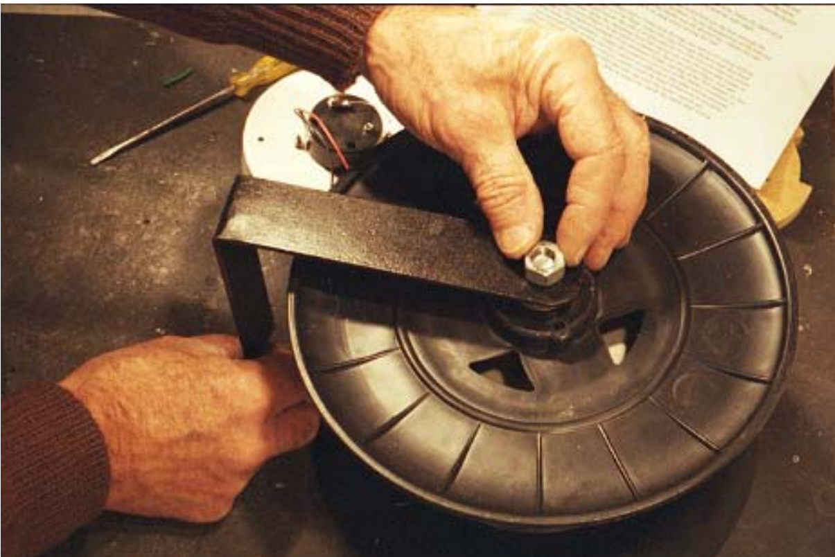
Figure 17. Attach handle nut.
