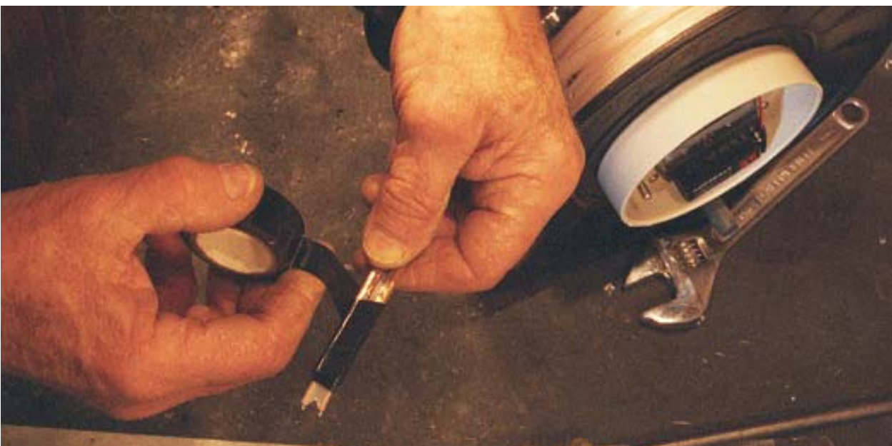
Figure 47. Wrap electrical tape around copper sheath.
