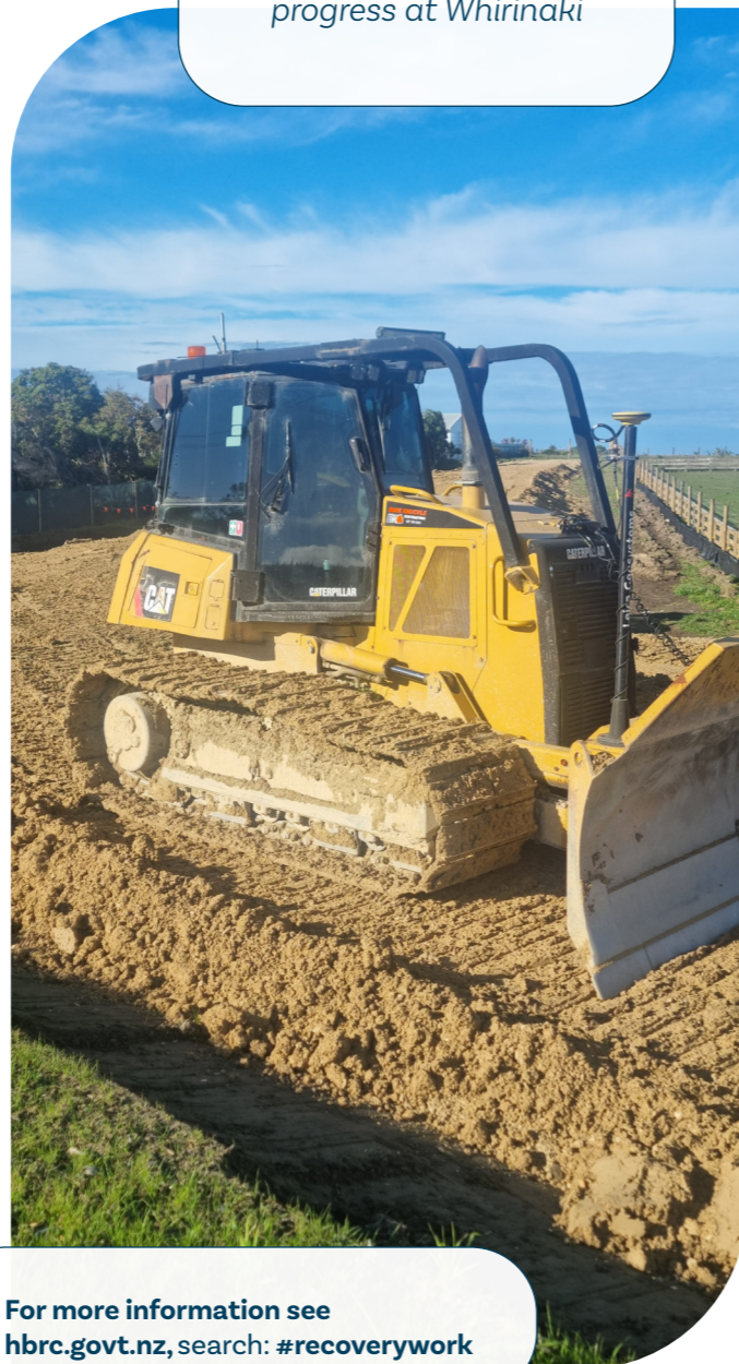
SH2 road raise and stopbank fill in progress at Whirinaki
