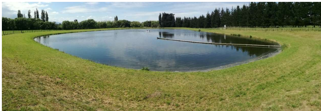
Figure 2 - Takapau WWTP Stabilization Pond
