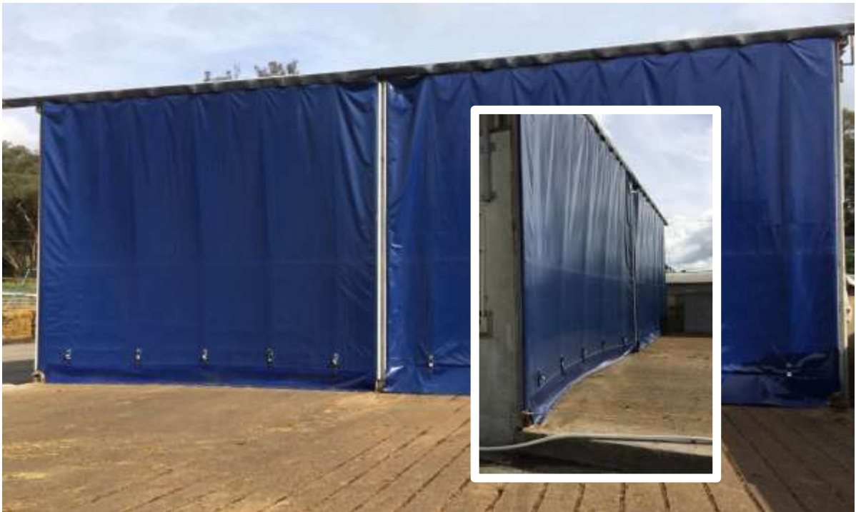
Bunker doors – closed. Insert shows side profile of same doors – with “bend” in the door walls from the vacuum suction internally. No gases observed escaping the bunkers.
