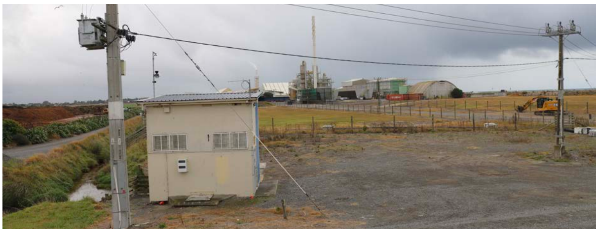
Figure 4: Pump Station Site – Looking North
