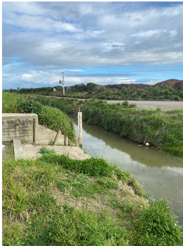
Photograph 4: The photograph is taken from beside the pump station building, looking west along the Mission drain.
