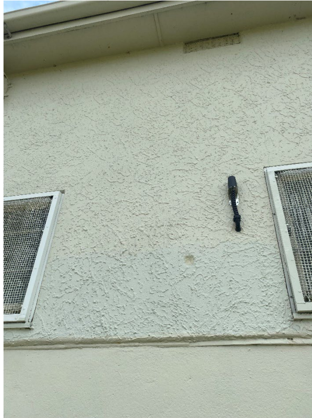
Photograph 3: The photograph is of the wall of the pump station building.
