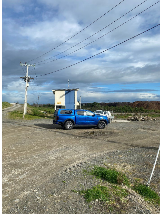
Photograph 1: The photograph is taken from the eastern section of the site looking west towards the pump station building, which can be seen behind the blue vehicle.
