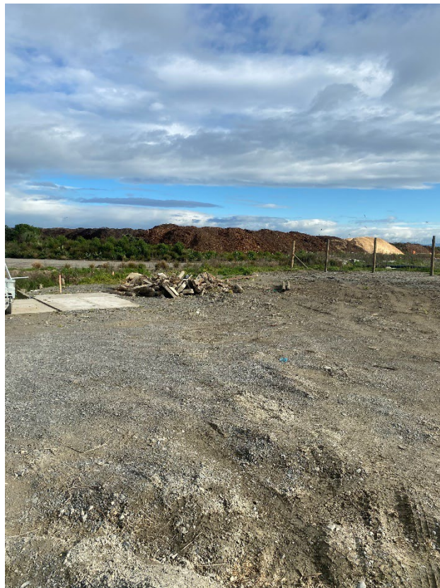
Photograph 8: The photograph is taken from beside the pump station building looking north-west. The clear area in the middle of the photograph is the area that was opened up to channel water from the drains to the river after Cyclone Gabrielle.
