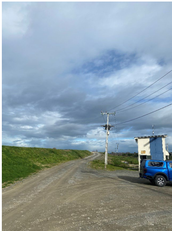
Photograph 2: The photograph is taken from the eastern section of the site looking west with the stopbank on the left and the pump station building on the right of the photograph.
