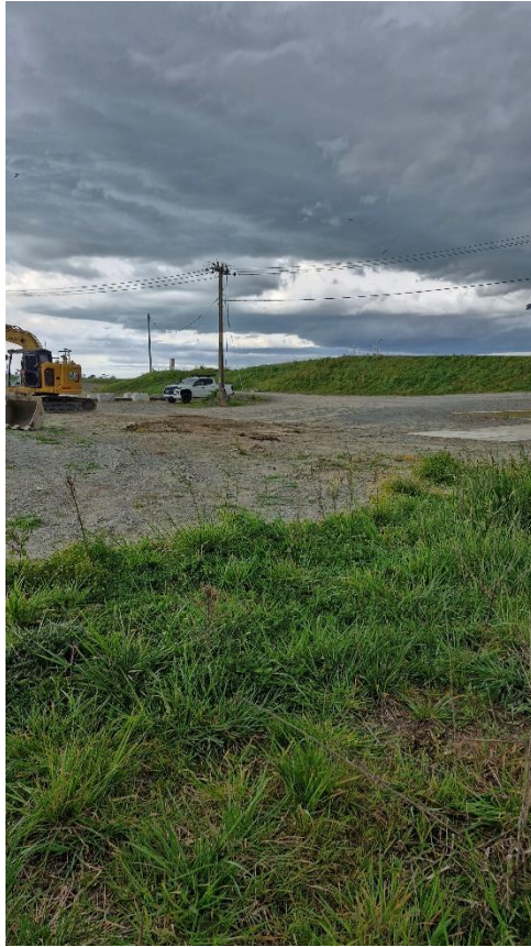
Photograph 3: View of the pumpstation access and carpark, facing southeast.
