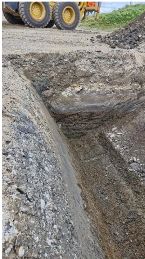
Photograph 6: View of test pit TP3 view, near pumpstation access, facing south.
