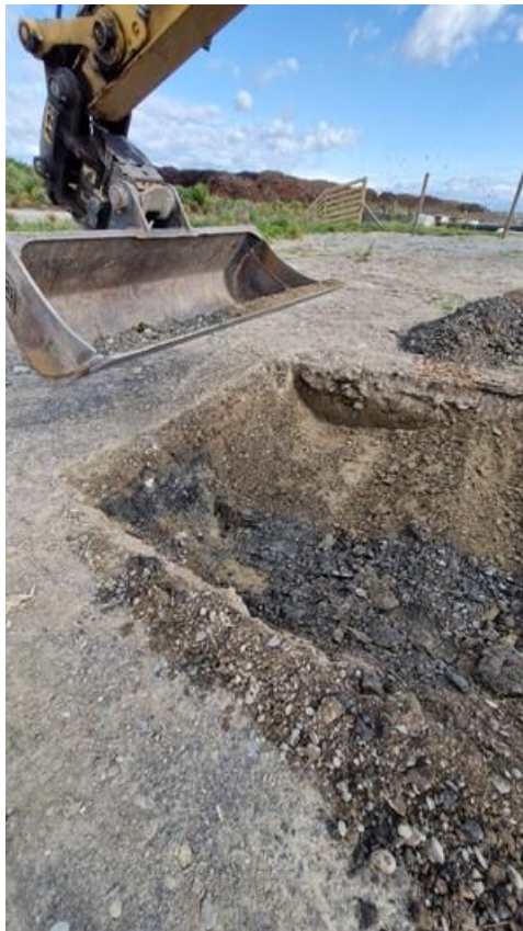
Photograph 4: Test pit TP1, near the pumpstation building, facing north.
