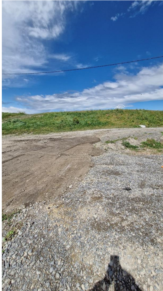
Photograph 7: Final state of test pit TP3 after reinstatement, facing south.
