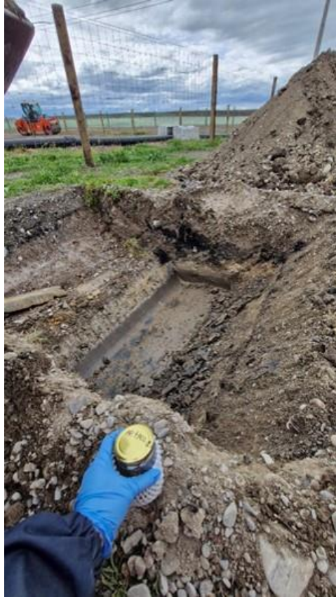
Photograph 5: View of test pit TP2, within the carpark, facing north.
