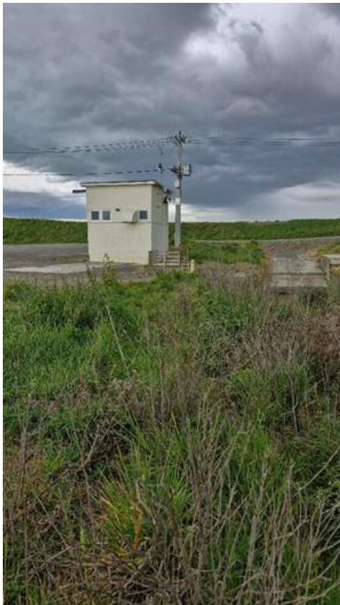
Photograph 2: View of the pumpstation's electric feed view, facing south toward the stopbank.
