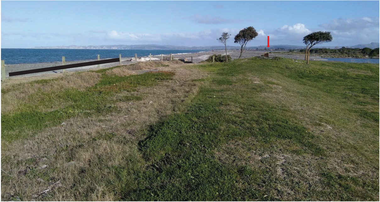
Figure 4 – The proposed access track (black line) and the location of the pillbox (red arrow).
