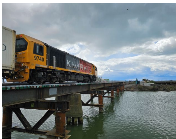
Figure 6: Completion of temporary bridge for Bridge 217 PNGL September 2023 (Source: TREC)
