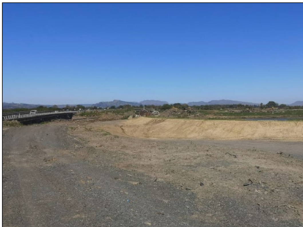
Figure 7: View of stopbank tie-in to Bridge 217 PNGL looking south (Source: Tonkin and Taylor – September 2023)
