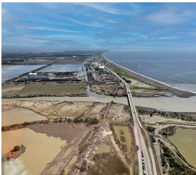
Figure 3: Aerial image of Bridge 217 PNGL post Cyclone Gabrielle (Source: TREC)
