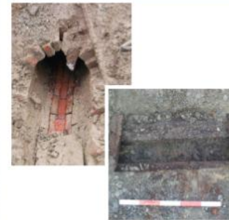
A 19th century drain made out of bricks (brick-barrel) and a timber box drain, used to keep the streets clear of water in the 19th century.
