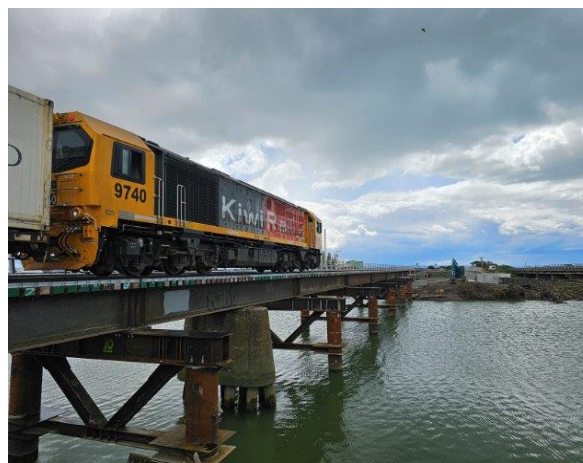
Figure 5: Completion of temporary bridge for Br 217 PNGL (Source: TREC)
