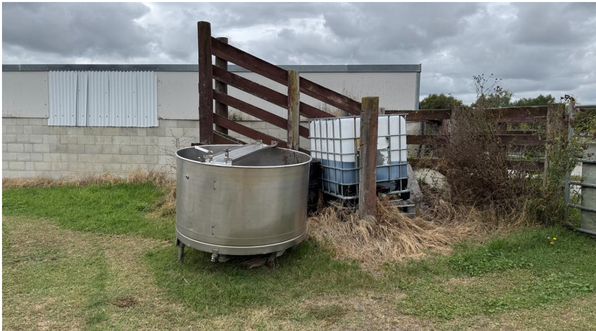
Photograph Appendix B.20: Suspected asbestos cladding on the milking shed at the rear of 131 Taihape Road on 28 February 2025. The suspected asbestos was observed to be in poor condition. An IBC with unknown dark coloured liquid is present near the gate in the left of the photograph.
