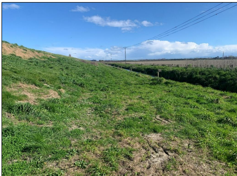
Figure 5 Stream berm habitat unit
