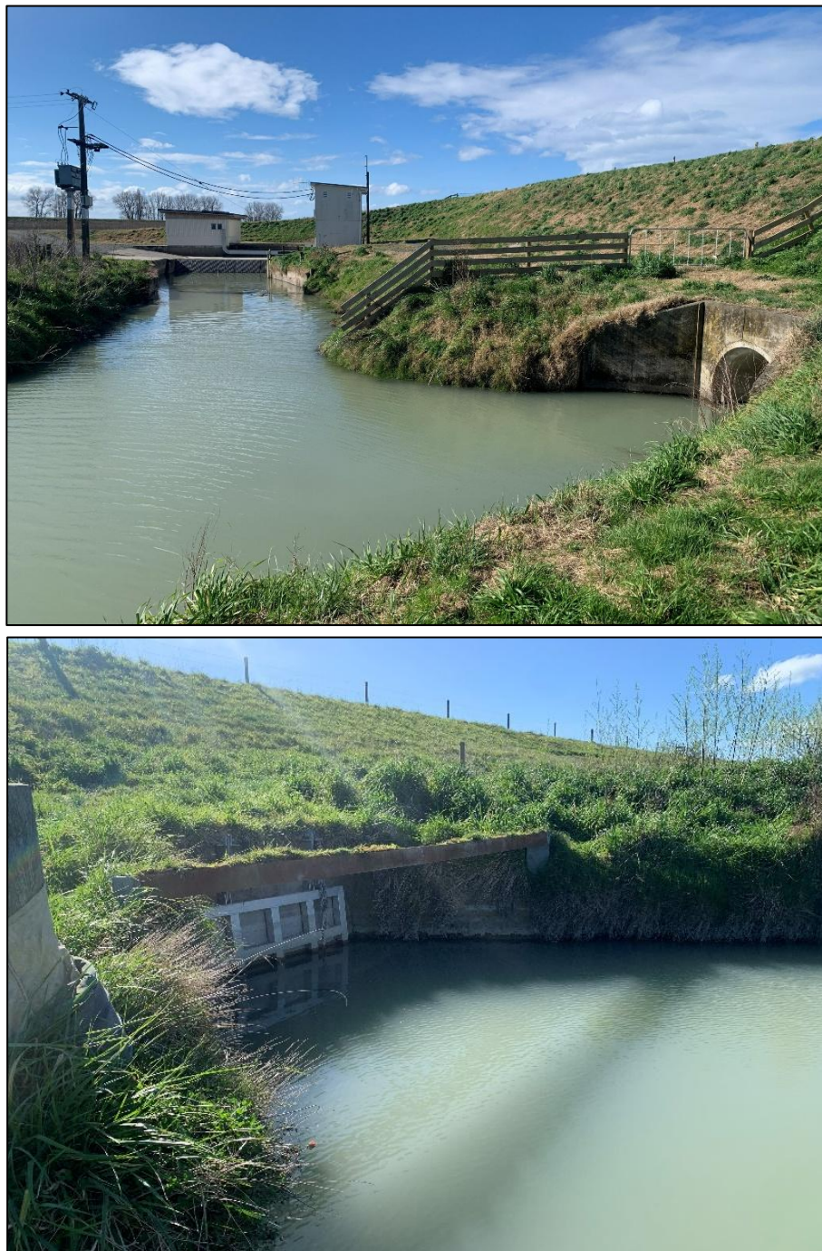
Figure 9. Gravity outflow upstream of Pākōwhai Pump Station. Top, the inlet side of the gravity flow bypass flowing to the right of image, with the existing Pump Station in background. Bottom, outlet side of gravity bypass, with conventional flap gate shut due to ambient river level.
