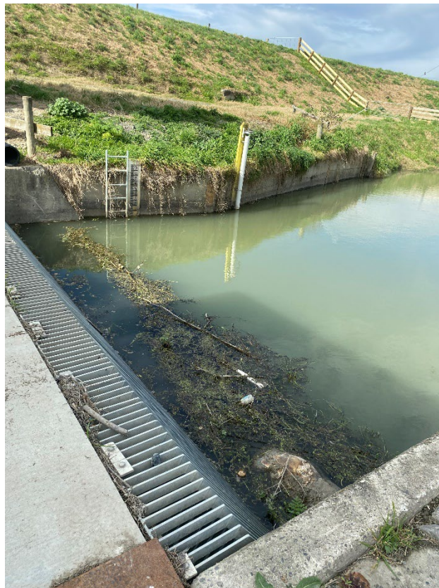
Photograph 4: View from the edge of the pump station's concrete slab, looking south-west along the main drain channel adjacent to the pump station.
