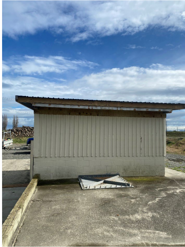
Photograph 3: View facing the western pump station building.
