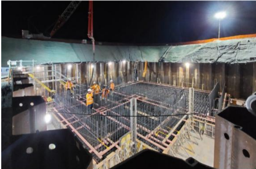
Example of working within a cofferdam, early morning concrete pour for pump station foundations
