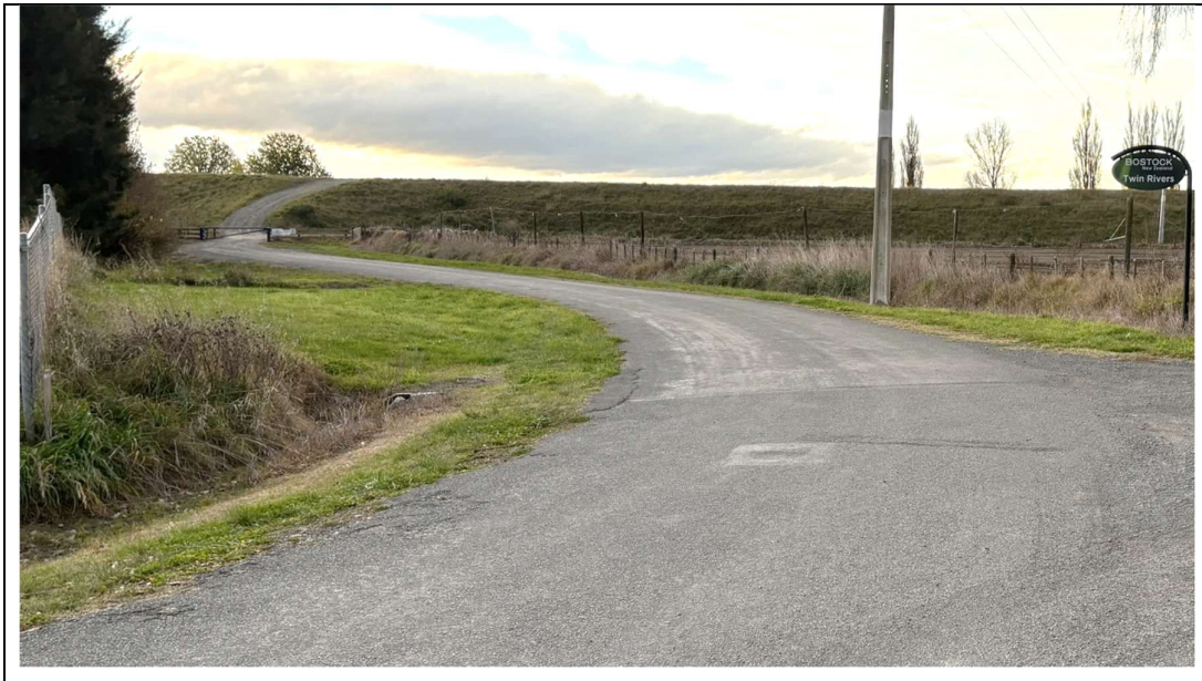
Figure 7 – Sissons Road narrow sealed section
