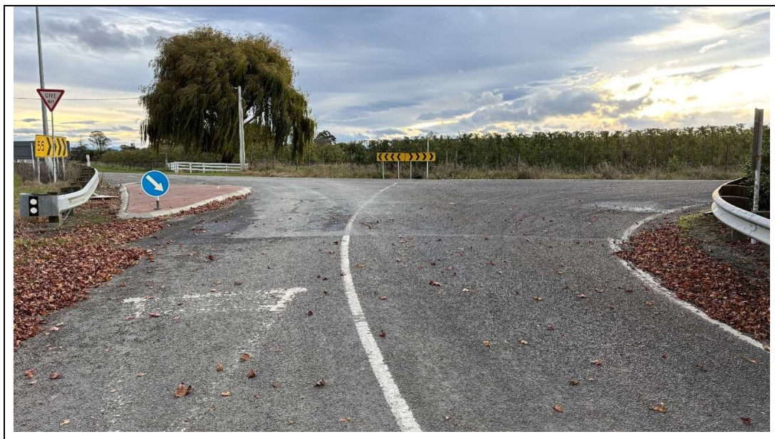
Figure 6 – Brookfields Road/Sissons Road Intersection
