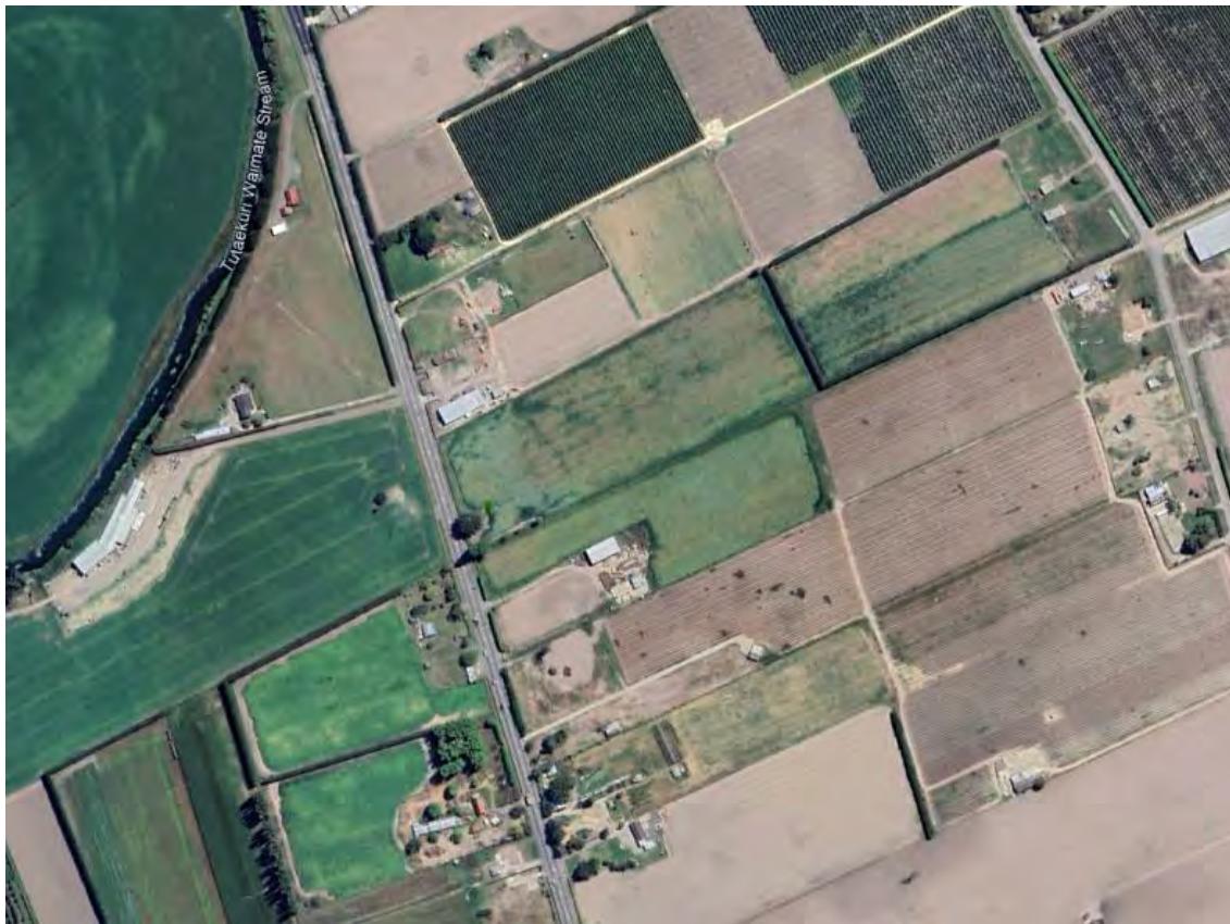
Figure 4.11: Latest aerial imagery downstream of proposed spillway (Google Earth, February 2025).
