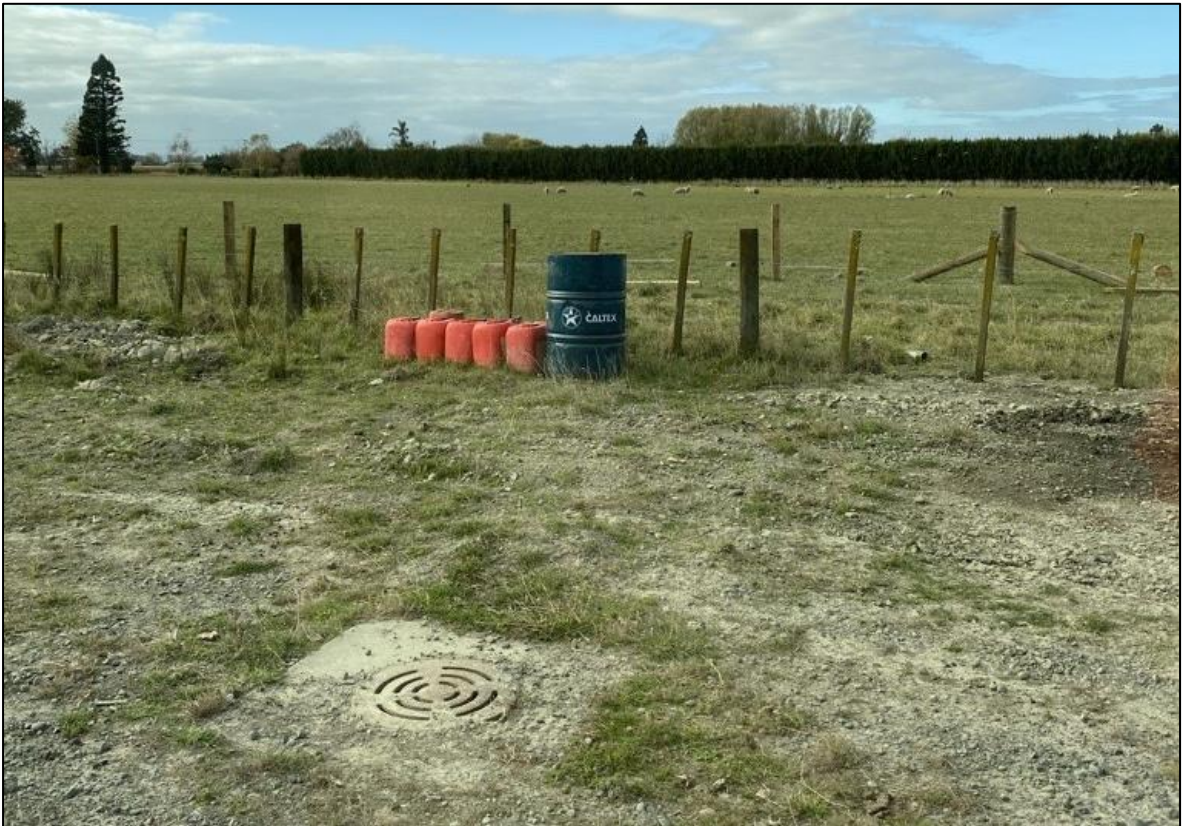
Photograph Appendix B.6: Drum and jerry cans (potential low-volume fuel storage) near to the damaged farm shed at 1854 Pakowhai Road.
