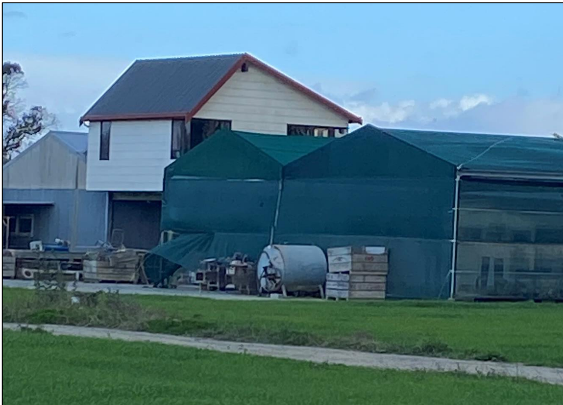
Photograph Appendix B.4: Aboveground storage tank (AST) at 43 Hodgson Road.
