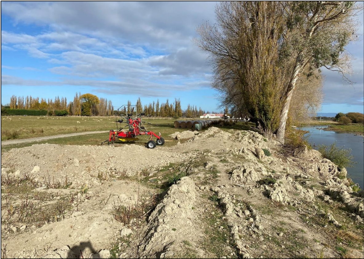
Photograph Appendix B.1: Silt stockpiles present along the Tūtaekurī Waimate Stream.
