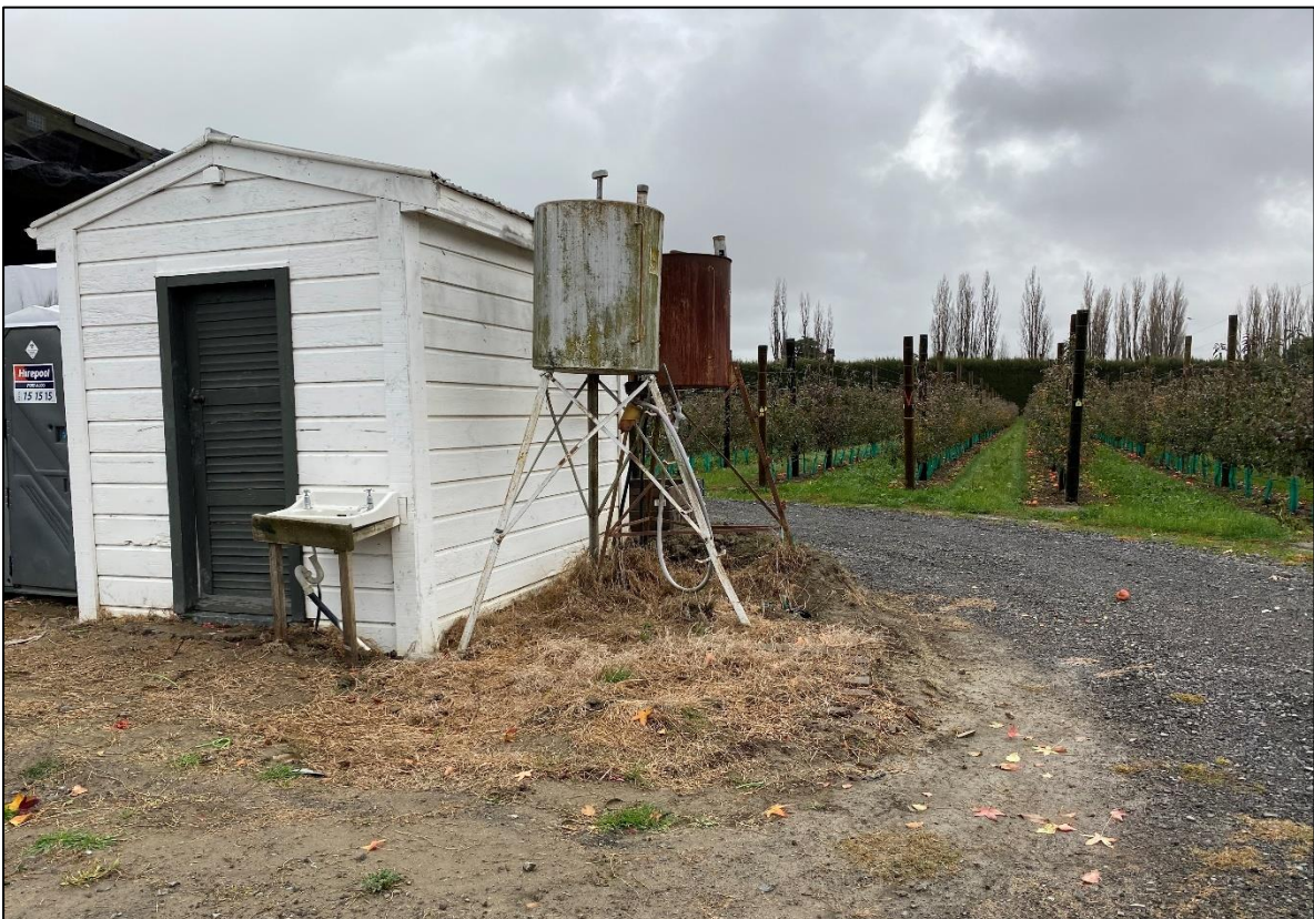
Photograph Appendix B.18: Two small AST's at 70 Franklin Road.
