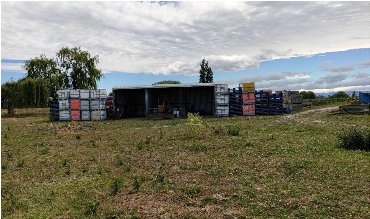
Photograph Appendix B.26: Site 7d – steel shed used for storage of machinery and farm equipment, with empty intermediate bulk containers and steel drums stored on either side.
