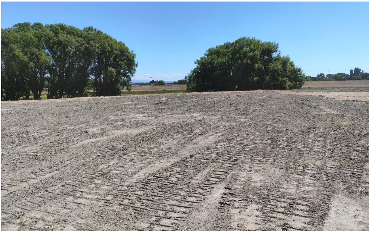
Photograph Appendix B.14: Site 4b – filled and graded paddocks, with trace refuse in loose soils. Facing north.
