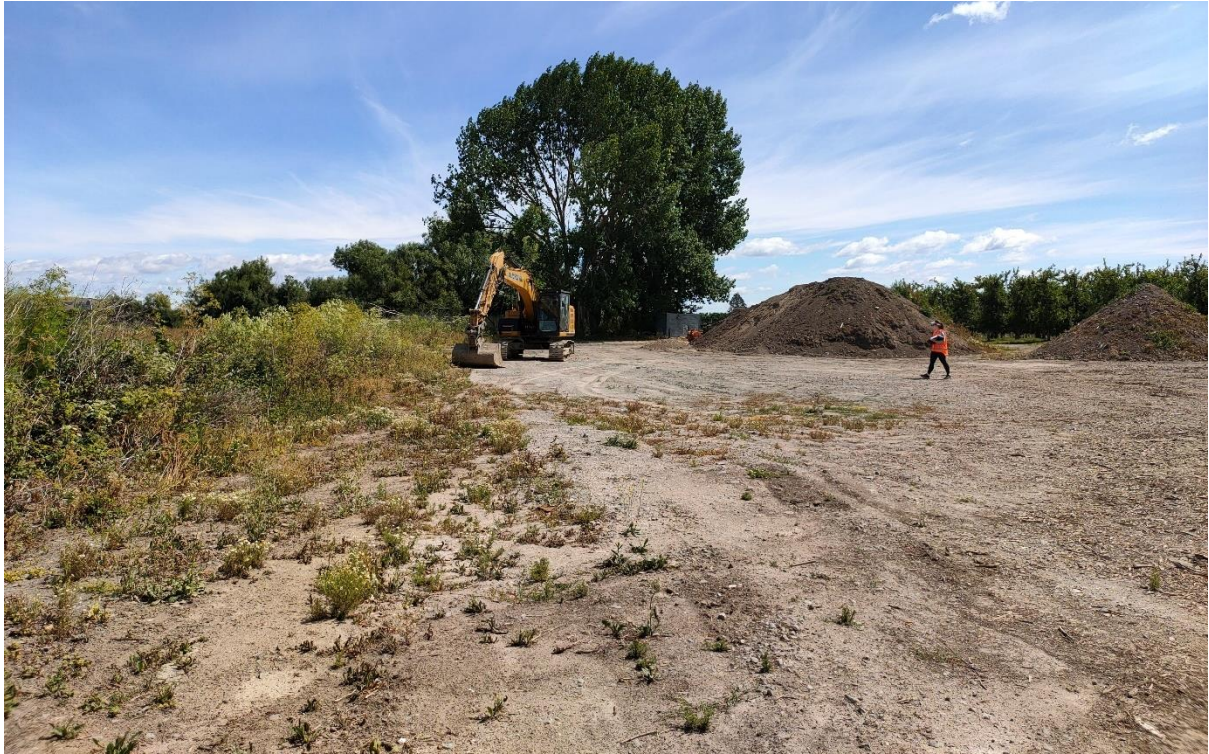
Photograph Appendix B.1: Site 1 – laydown area with stockpiled soils. Facing north.
