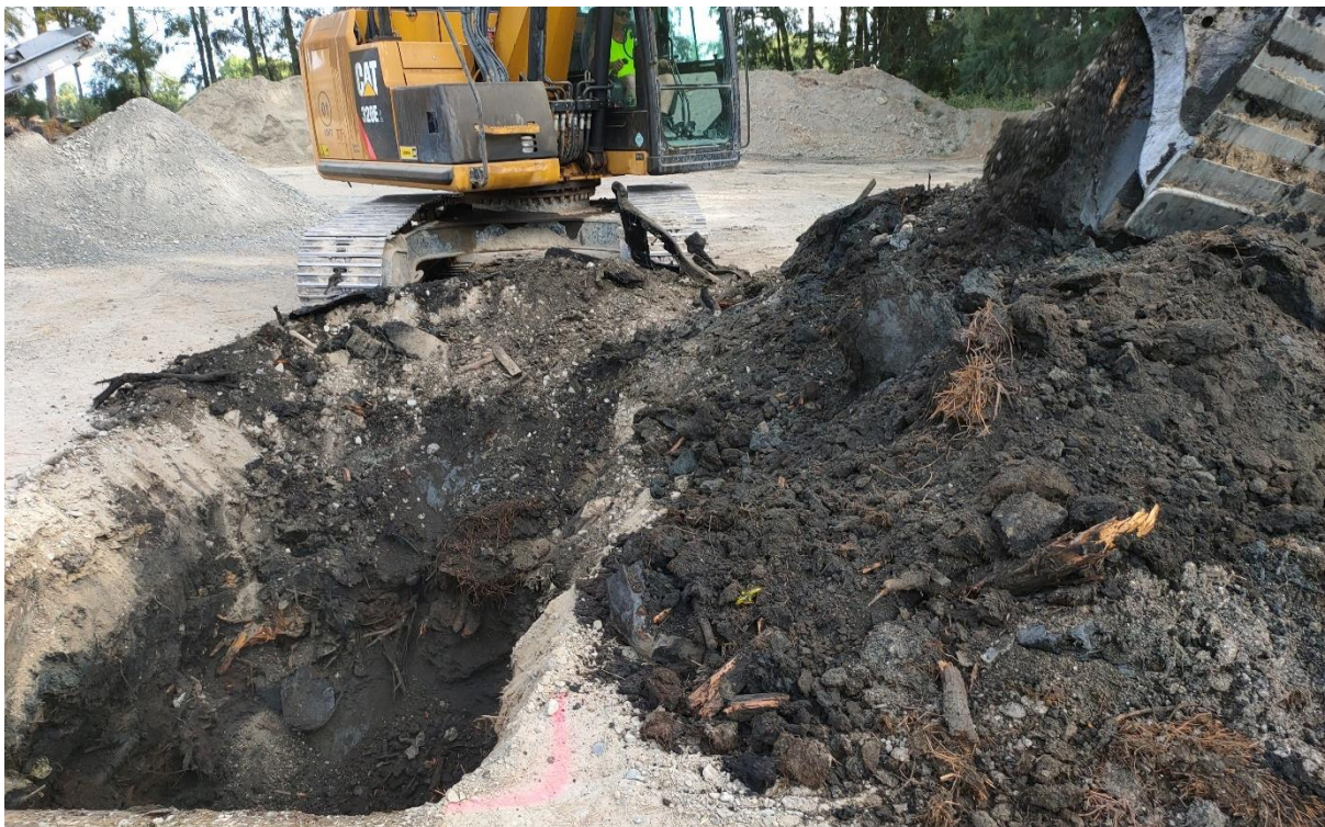
Photograph Appendix B.8: Site 2 – Large volumes of organic material and industrial waste in S2_TP6.
