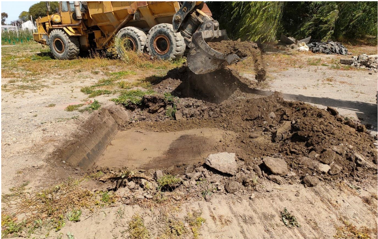
Photograph Appendix B.4: Site 1 – natural soils in S1_TP4 at southern end of site.
