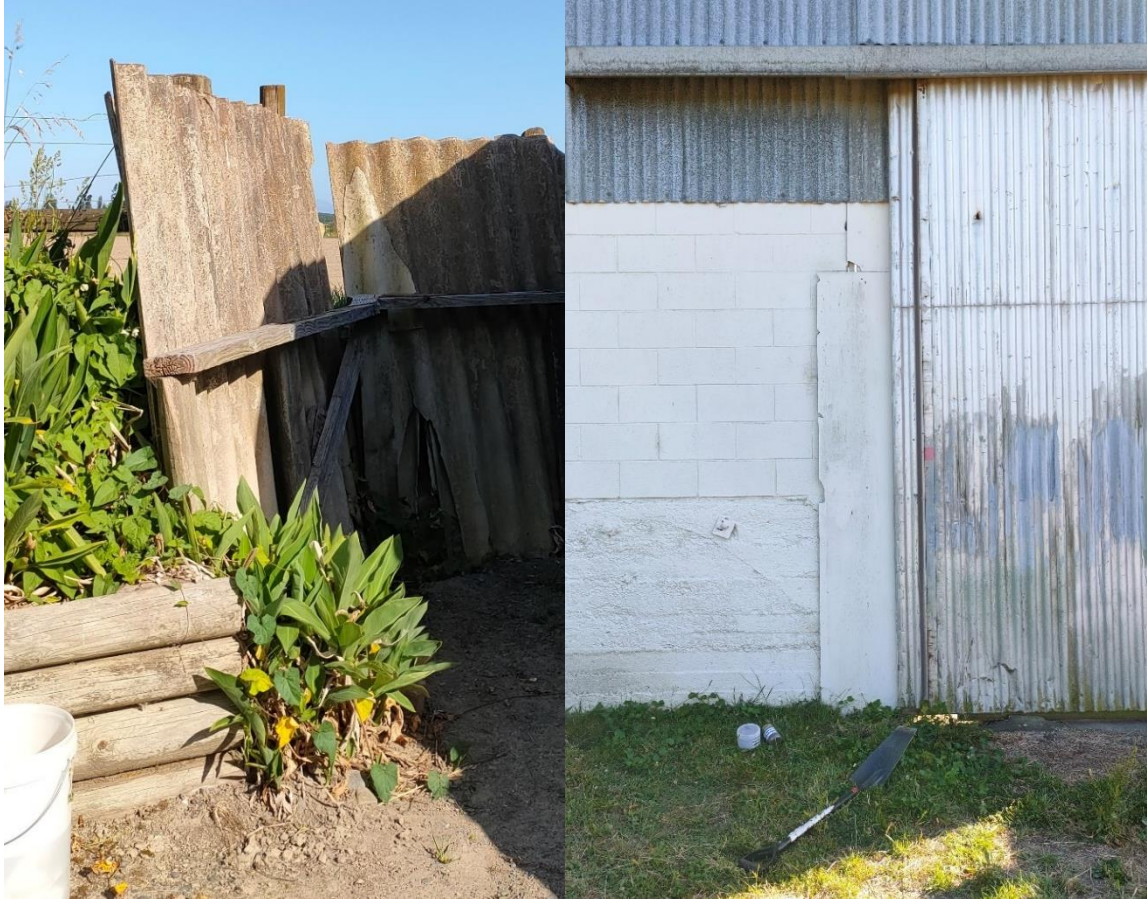
Photograph Appendix B.25: and 25B: Site 7c – suspected ACM products at 22 Chesterhope Road. ‘Super 6’ fencing (left) and fibre board in tack shed (right).
