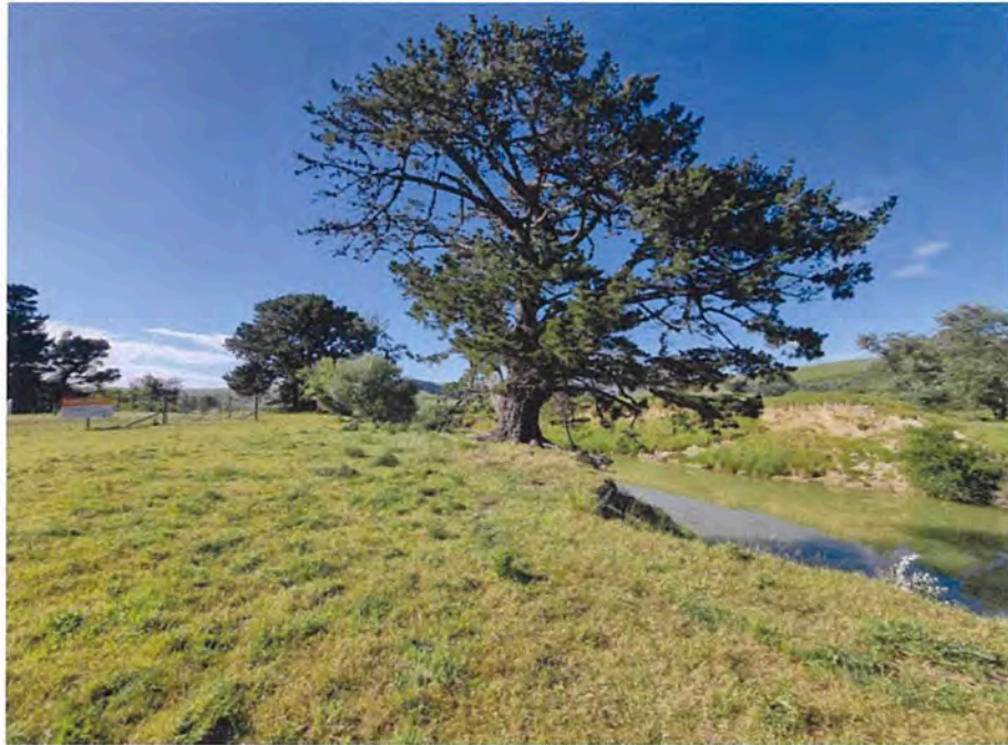
Photograph 1: Properties A and B - The photograph is taken from the northern side of the river looking downstream. The wastewater pond is located behind the sign and fence near the middle left of the photograph.
