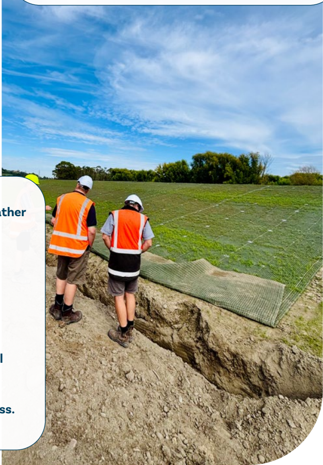
Ground and cycle trail being reinstated at the Waiohiki stopbank
