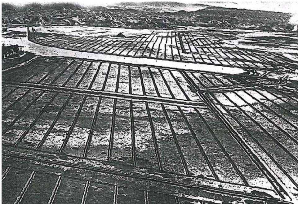
Figure 1-3: Drainage channels constructed to the north and south of the main estuary outfall channel to develop agricultural land. Source: Hawke's Bay Museum.
