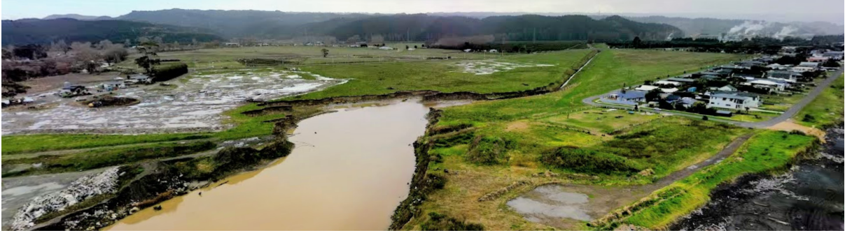
Figure 3: Aerial view of the southern end of the project area.
