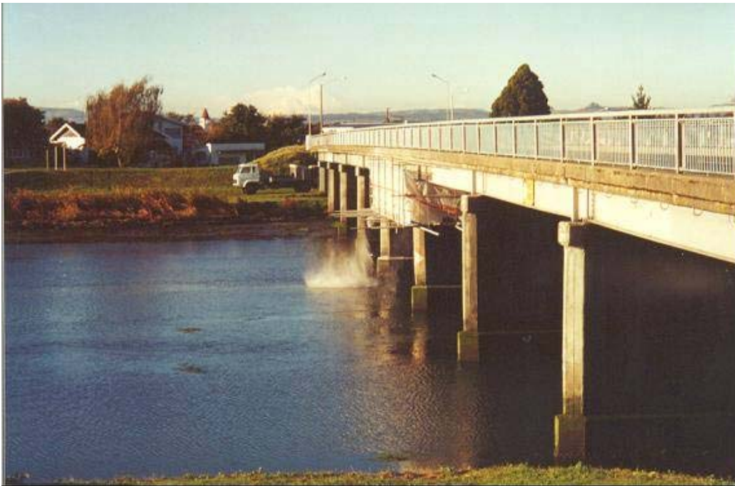
Figure 5.: Illustration of dust impacts of sandblasting a bridge in the Hawke's Bay Region (photo supplied by Bryce Lawrence, HBRC)
