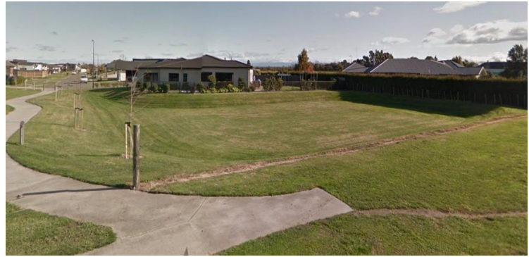
The Lyndhurst development has detention ponds that double as park and play areas.
