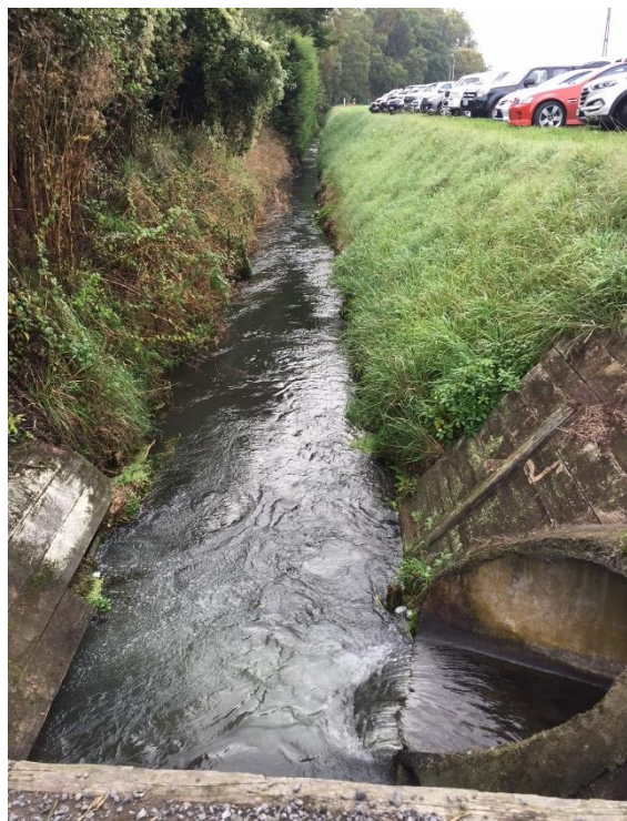
The 'Unnamed Drain' (bottom right) contributes spring-fed flow to Raupare Stream. Raupare Stream flows at a rate of 300 litres per second through a tile drain created in the 1920s.
