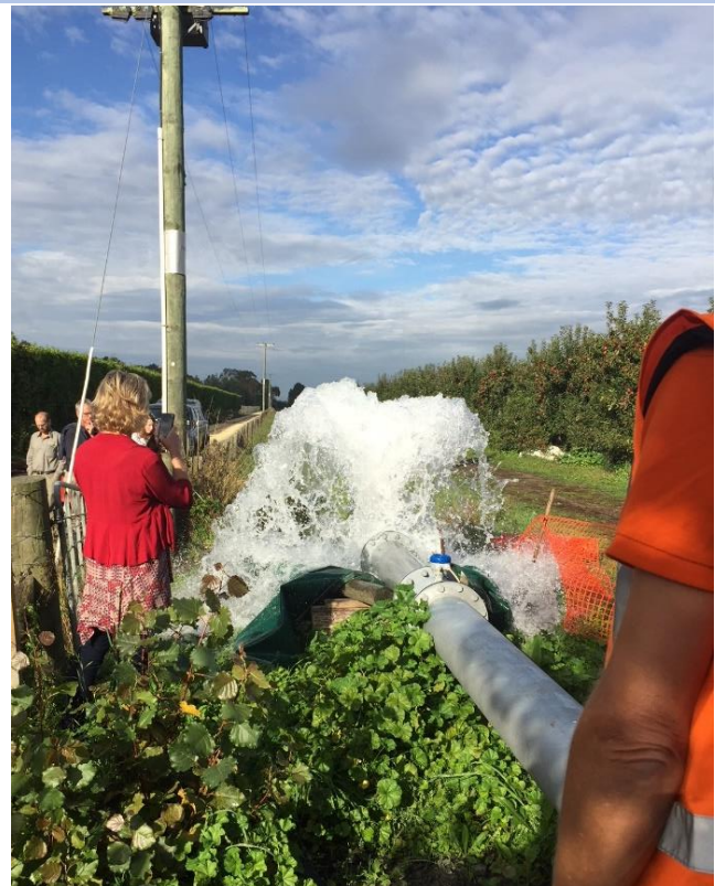
Impressive when it's in action! This new augmentation structure is one of 2 in place in Twyford, to augment flow to Raupare Stream.
