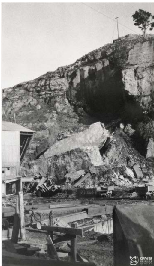
Figure 1.1 Rockfall at Ahuriri caused by the Hawke's Bay Earthquake in 1931 (GNS Science).
