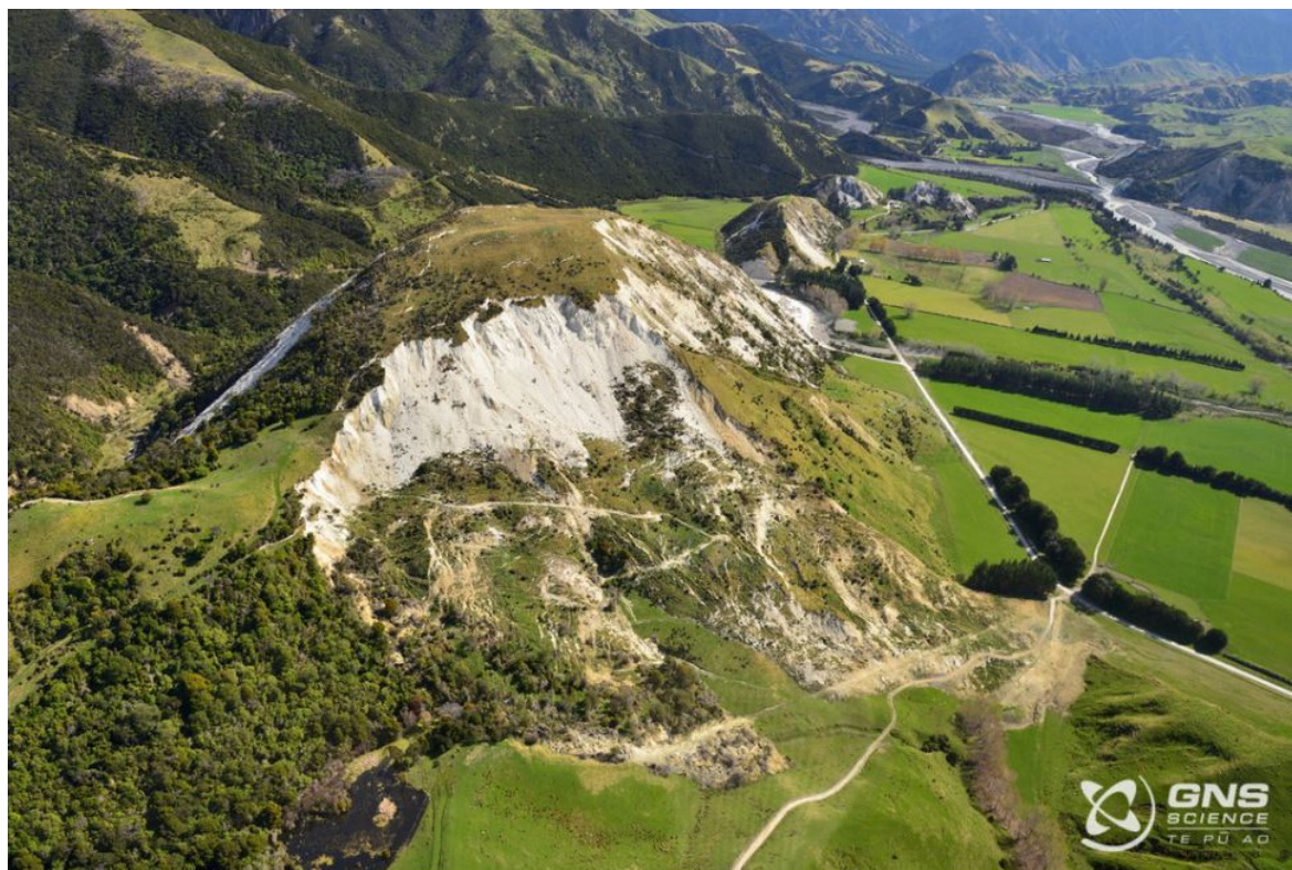
Figure 1.3 Debris flowslide resulting from the rupture of the Papatea Fault near Clarence River following the 2016 Kaikōura Earthquake (GNS Science).
