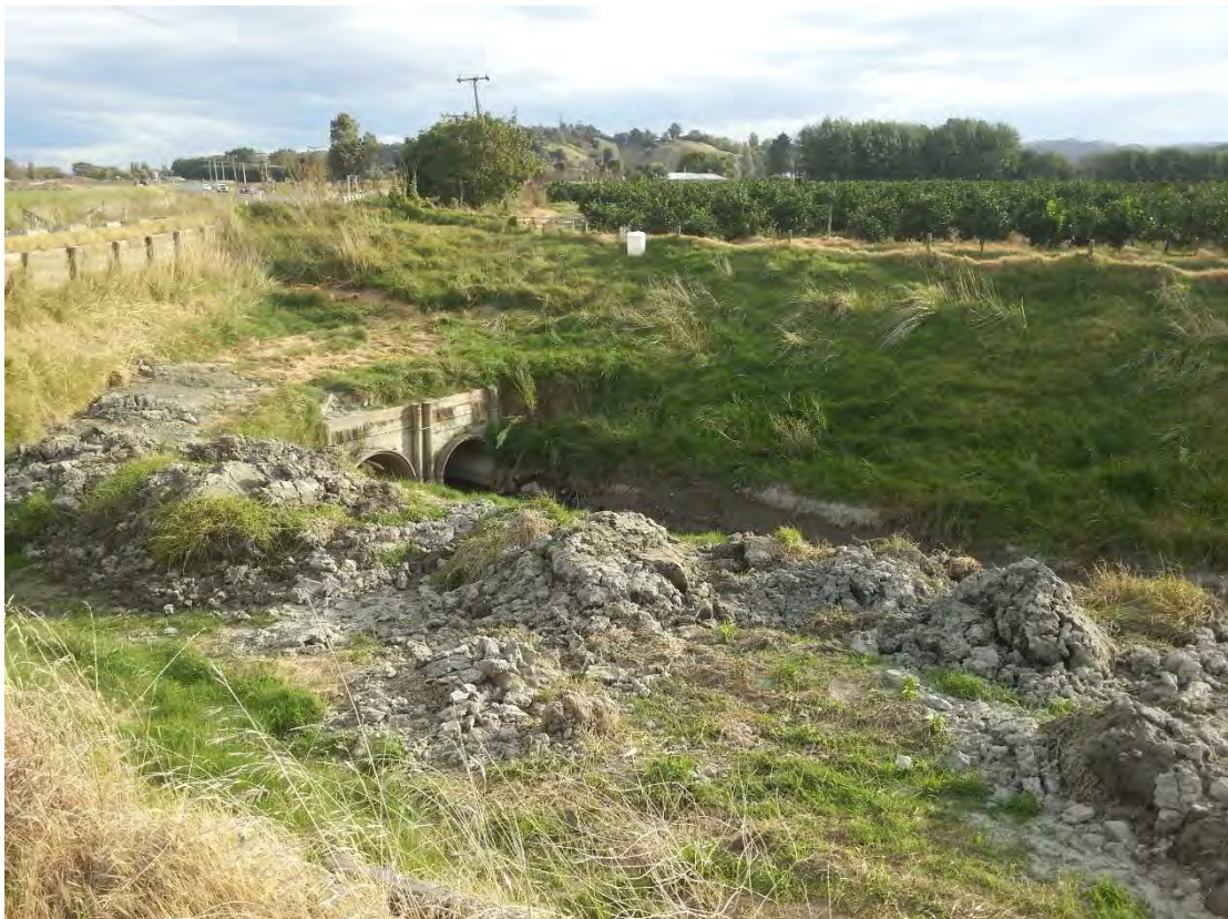
Photograph 12: Whirinaki Drain looking south at the culvert under SH2 on 27 March 2024. The site is in the foreground with the visible piles of soil/sediment.
