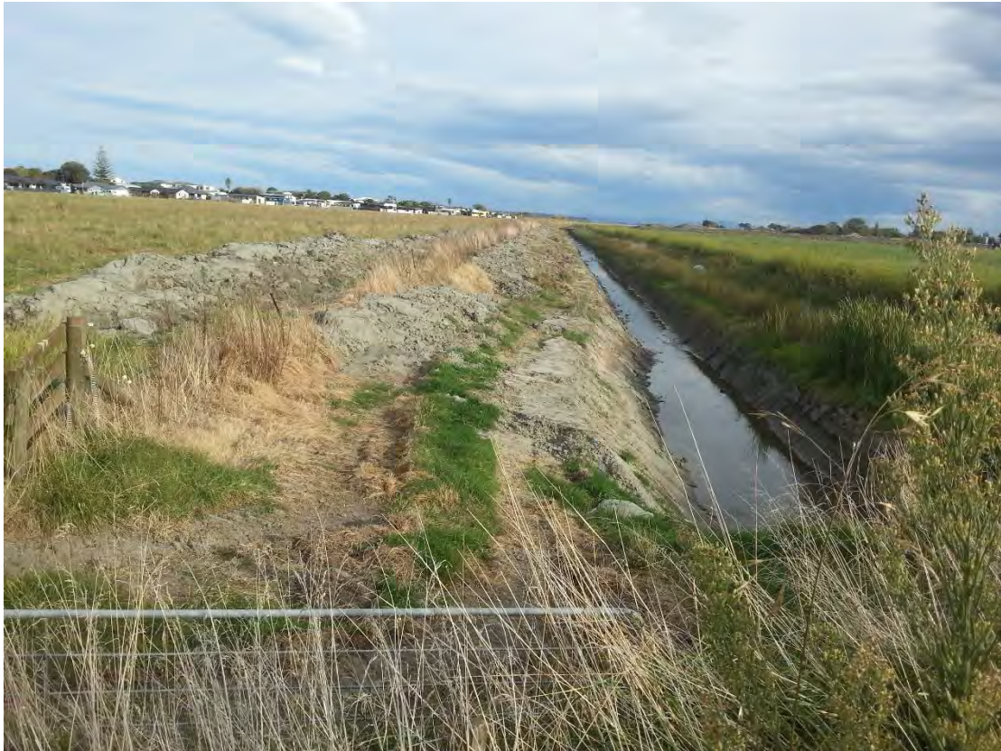
Photograph 11: Whirinaki Drain looking south towards the ocean on 27 March 2024. The site is along the left side (east) of the drain.
