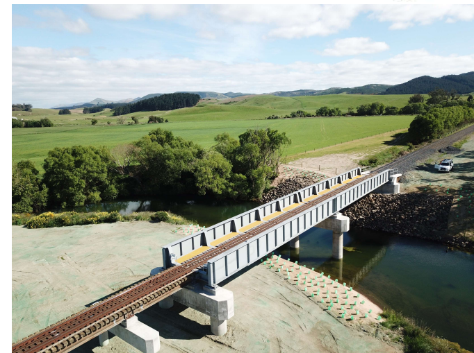
Steel Direct Fixed Span
