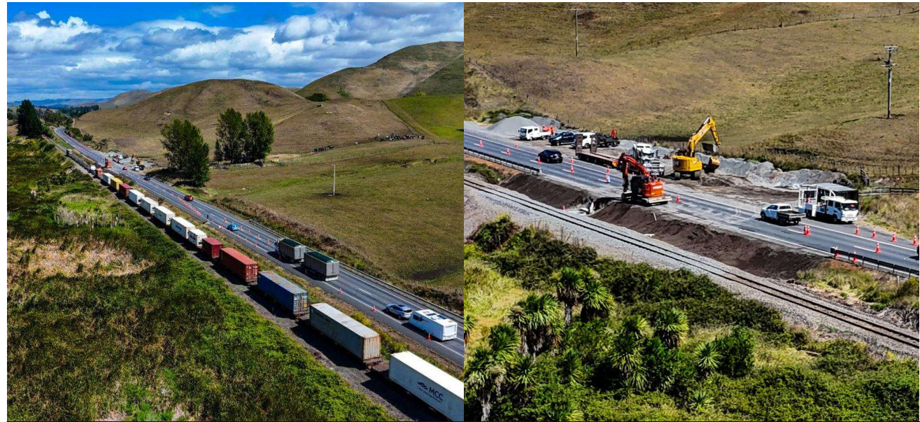
Pakipaki rail site, managing trains and state highway traffic
