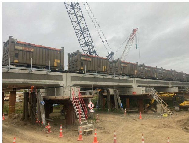
Concrete Ballast Deck Span
