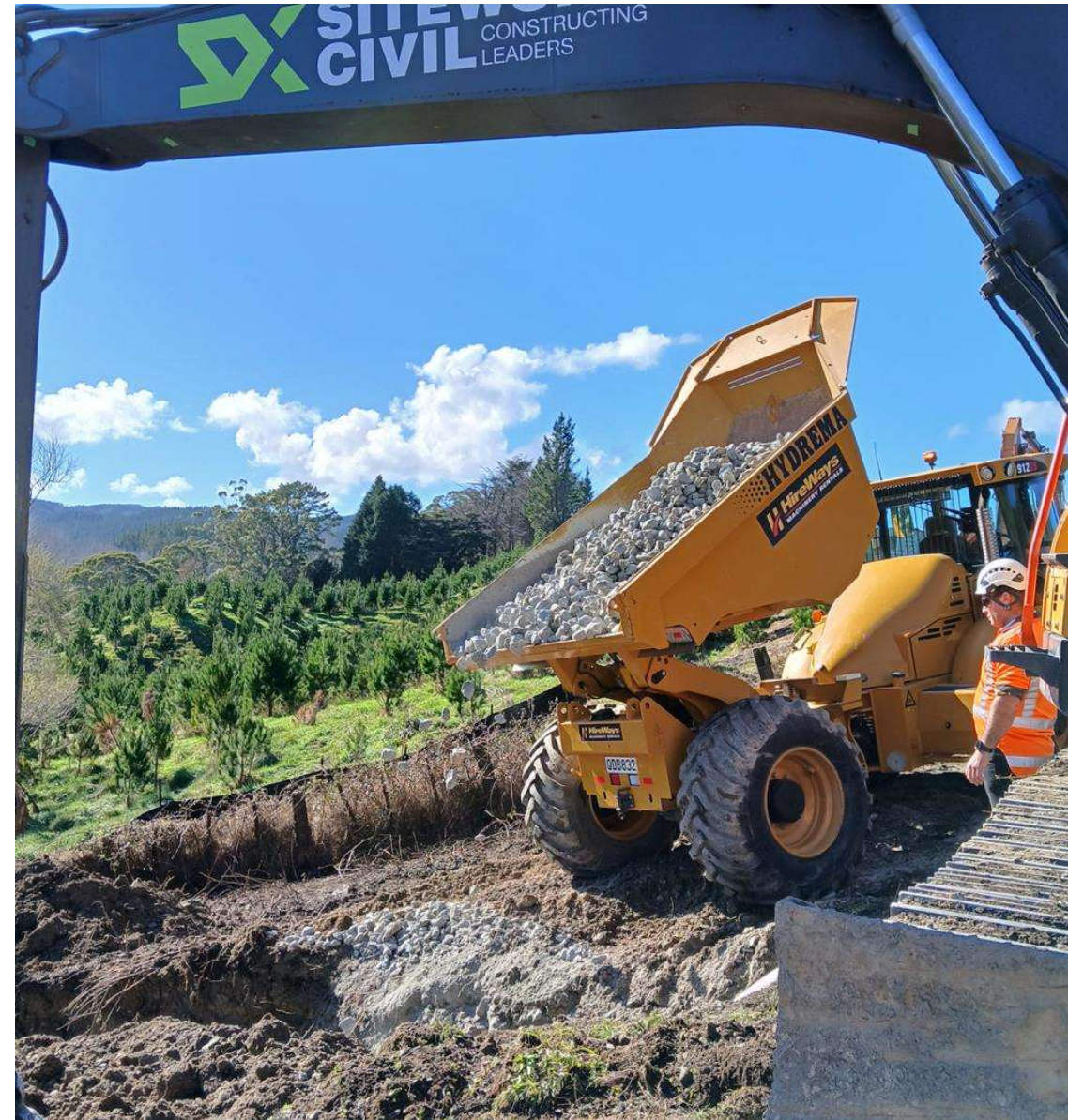
North Mōrere underslip repairs
